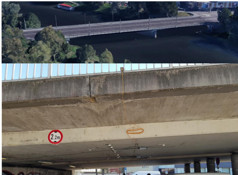
Fig. 1. Two bridge pilot applications, (top) Wonka bridge, Pardubice, Czechia, (bottom) Vogelsang bridge, Esslingen, Germany showing also the monitoring strain gauges.
