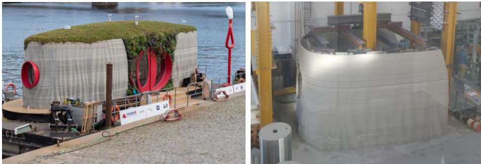
Fig. 8. Final view of the 3D printed building and its laboratory load testing.
