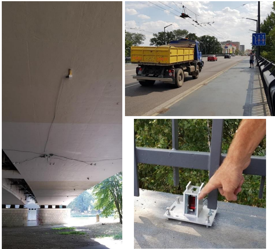
Fig. 2. Typical arrangement of iBWIM monitoring system installed on an investigated bridge (left) a calibration truck crossing the bridge (top right), and a laser sensor for the detection of the passing vehicles and number of axles (bottom right).
